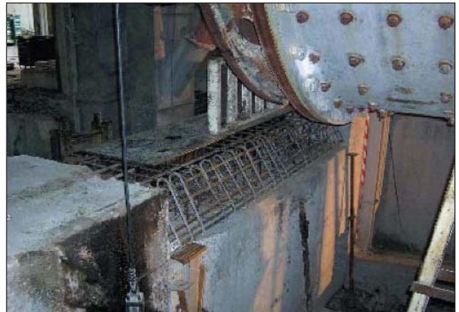
Figure 2. Mill exit side foundation.
