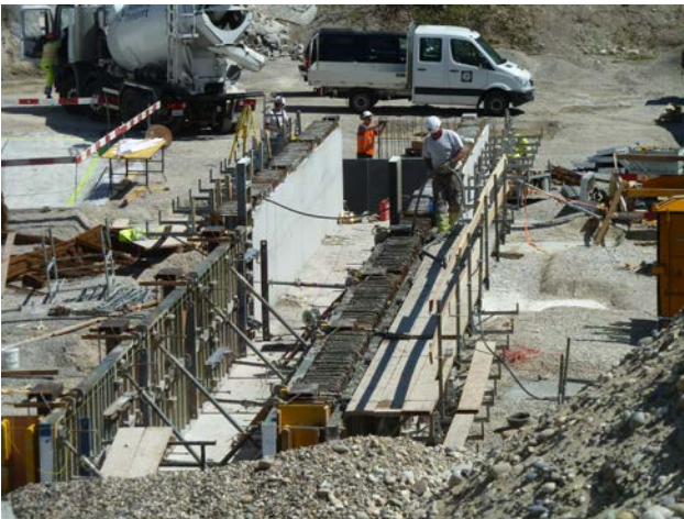
Foundation for pocket silos
