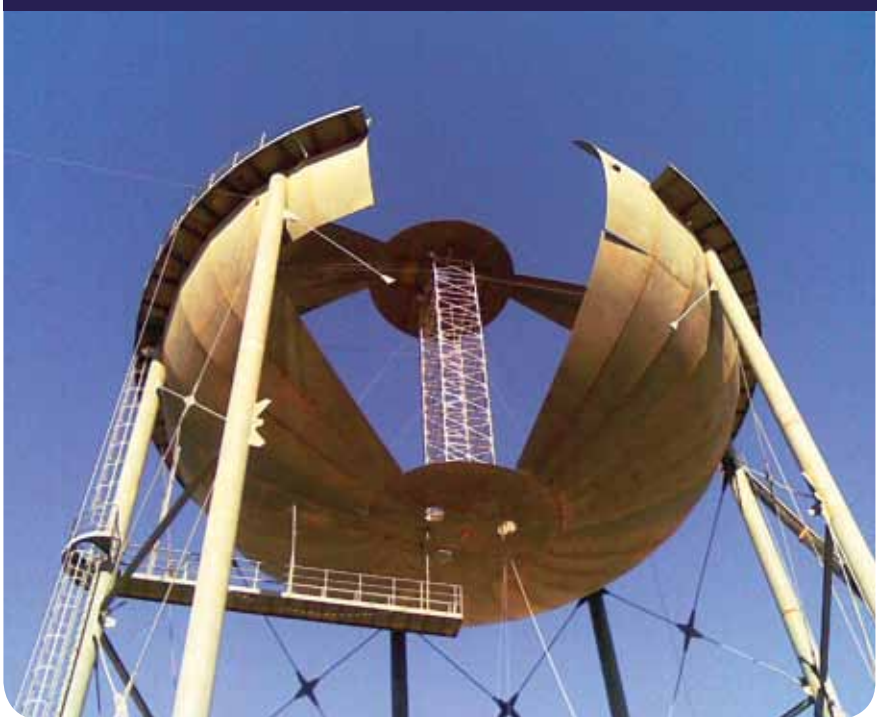
A positive example of economic, smart design and good designer-peer reviewer collaboration: an elevated water storage tank for a water treatment plant in Iraq, supplied by a specialised company
