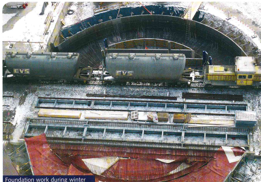
Foundation work during winter
