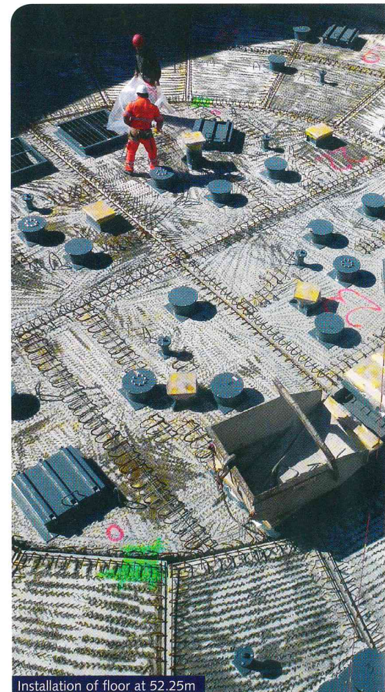
Installation of floor at 52.25m
