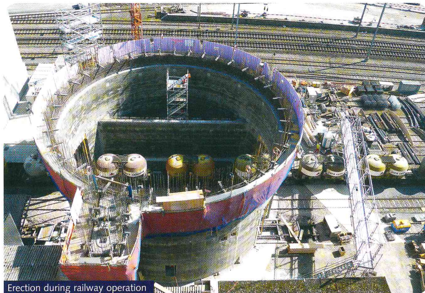
Erection during railway operation
