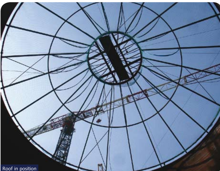
Roof in position
