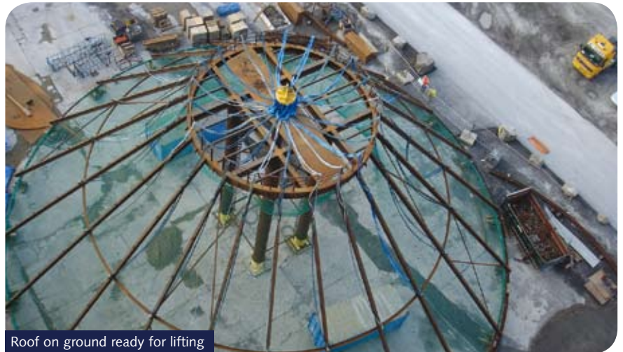
Roof on ground ready for lifting
